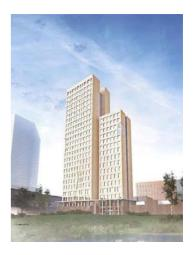
Roughly 3,600 m3 of wood are used in the entire construction, corresponding to 0.6 per mill of Austria's annual surplus timber production.
